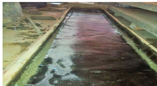
Figure 3. Internal wrapping
